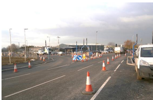
New filter lane at Watercombe Lane/Lysander Junction
