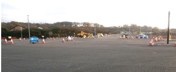
The transformation of the Lysander Roundabout to a signal-controlled junction nears completion
